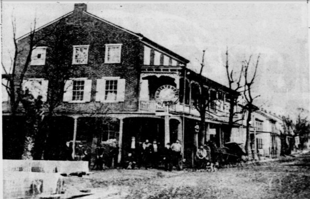
LOCAL LANDMARK — Filbert's Hotel, on the corner of Main and Goodman streets in Strausstown, is shown in this photo dating from some 70 years ago. Built by Jacob Boltz in 1845, the structure served as a public house until it closed in 1969. The porches had long since been removed.
