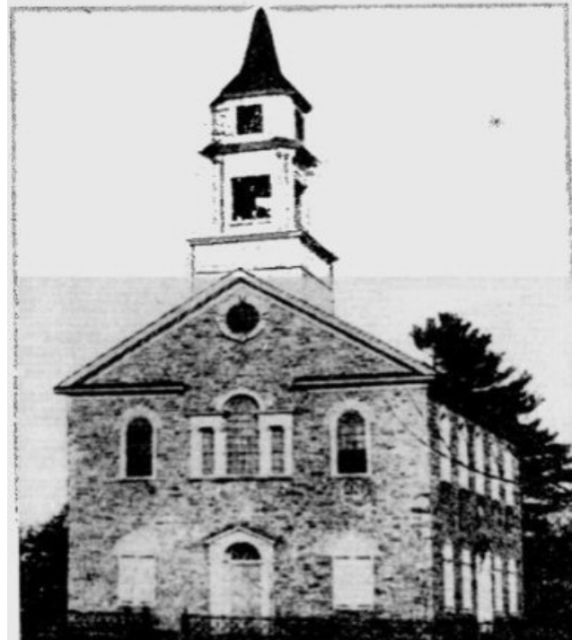
RAZED — The old Zion (Blue Mountain) Church, just east of Strausstown, stood from 1819 until replaced by a new edifice in 1904. It had ornate entrances on three sides and contained a Dieffenbach organ. This was a union church building, serving both the then-Reformed and Lutheran congregations. — Photos from the collection of George M. Meiser IX.
